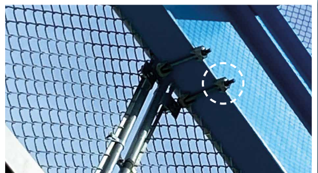
Type CF clamps used with threaded rod to connect the straps
