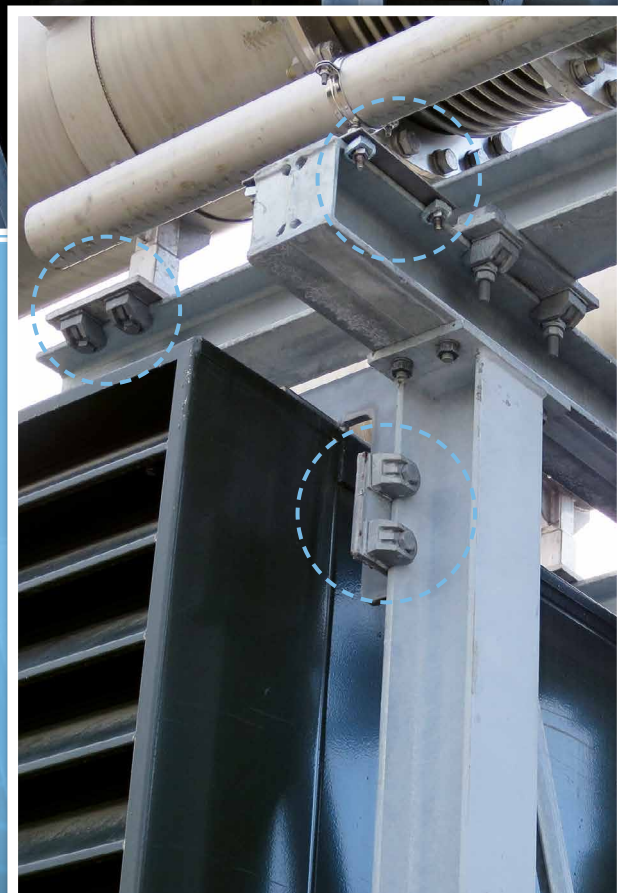
Girder Clamps used for tensile & frictional connections
