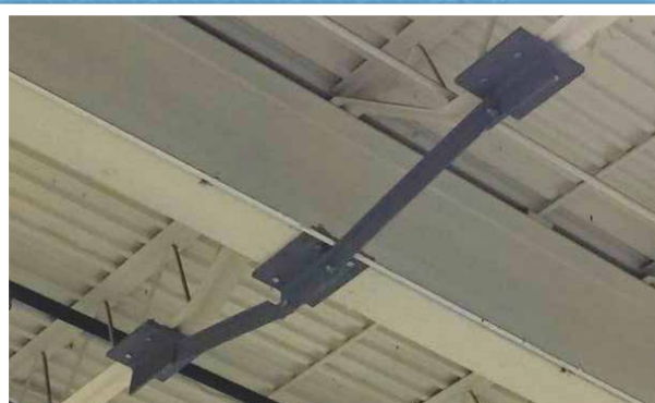
Type AF Girder Clamps connect the bracing support
