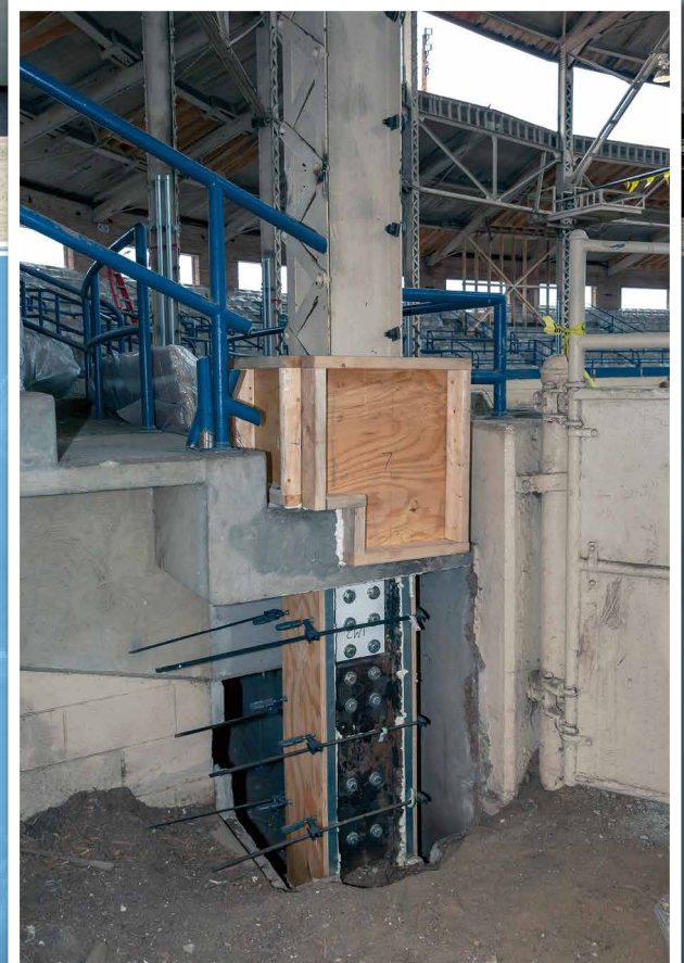
Hollo-Bolts connected reinforcement plates to the columns
