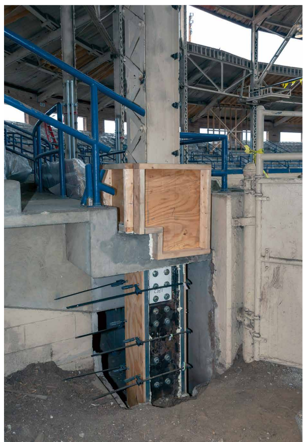
Hollo-Bolts connected reinforcement plates to the columns
