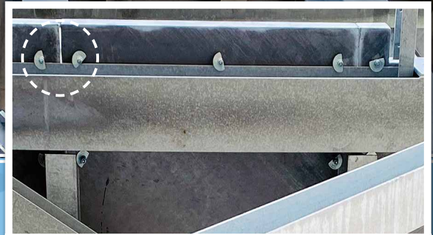
FloorFast installed underneath the finished floor
