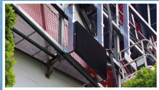
Installers tightened the Lindapter clamps on the plate brackets to the existing frame on the bunker
