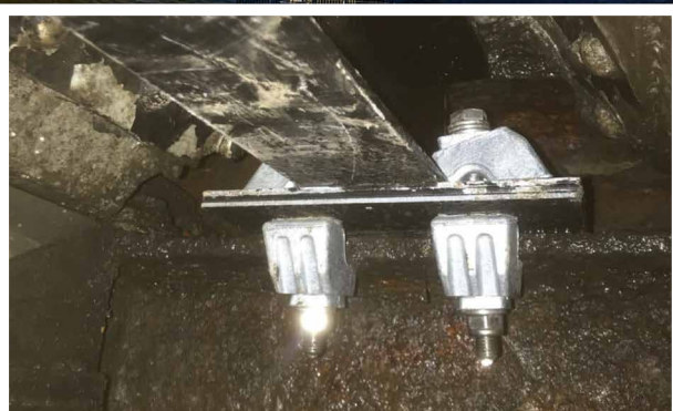
Type AAFs used to connect bracing support beams
