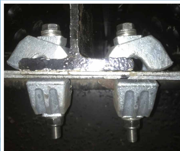
Girder Clamps provided a drilling and weld free connection
