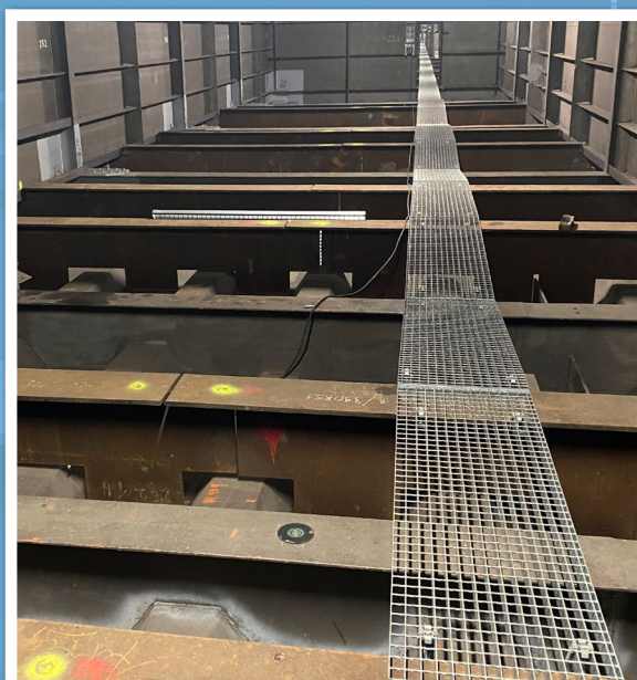
Steel bracing struts installed inside and along the length of one steel box section
