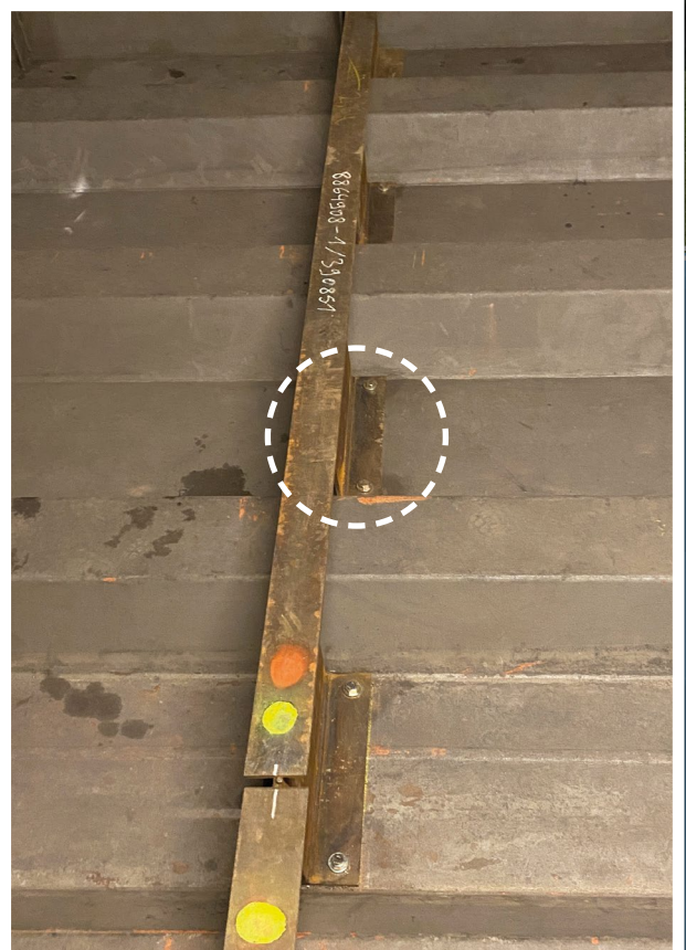
Steel bracing struts connected to the base of the box sections with Hollo-Bolt
