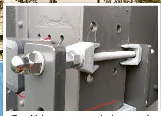
Type CF clamps provided a reliable, adjustable attachment point for the safety rope brackets
