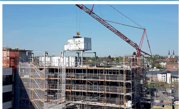
Air conditioning units being installed
