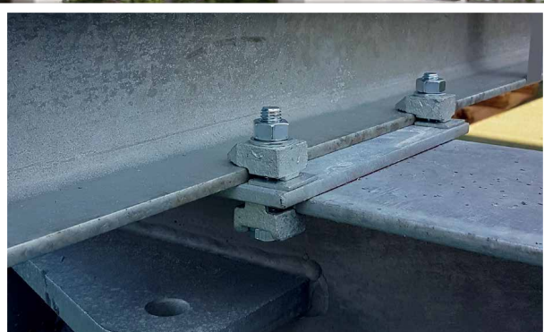
Girder Clamps connect the steel framework
