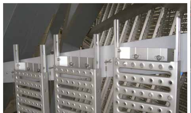
Hollo-Bolts connect the cladding panel brackets
