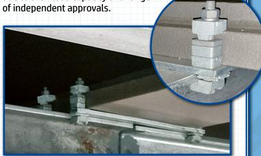
The client was concerned that clamps could become loose overtime due to the vibrations caused by the trams on the bridge deck above, and the additional cost of maintenance if they had to go under the bridge to retighten them. To provide extra reassurance and for a "belt and braces" approach anti-vibration washers were specified, Lindapter are the only manufacturer to have ETA approval for the use of anti-vibration washers with girder clamps.
