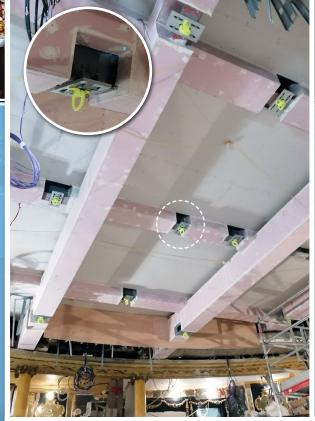
Lindapter's adjustable lifting point solution ensured minimal disruption to the existing structure
