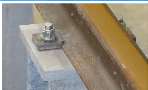
Type HD rail clips used to secure the rails
