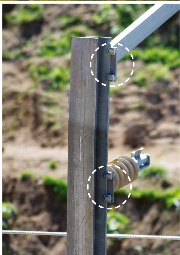
Type A girder clamps secured cantilevered arms to steel columns & OLE insulators to I-Beam masts
