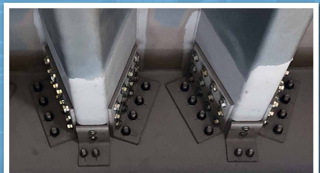
Hollo-Bolts provide an approved solution for dynamic load applications
