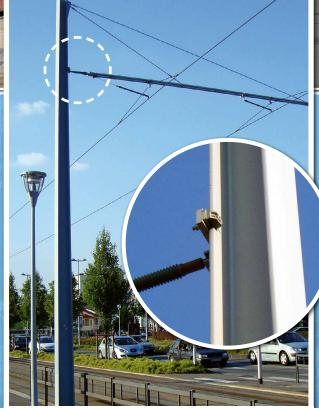
Type AF girder clamps connect cantilevered support arms to steel masts
