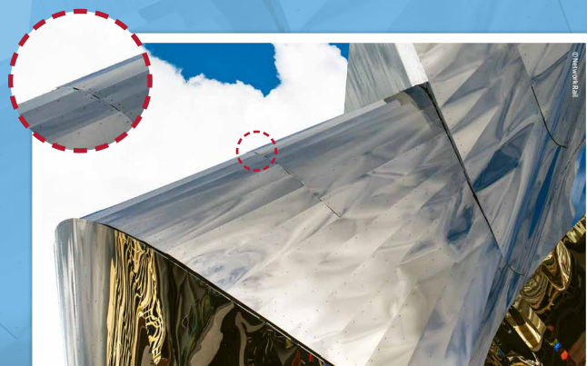
Countersunk head provided a neat finish
