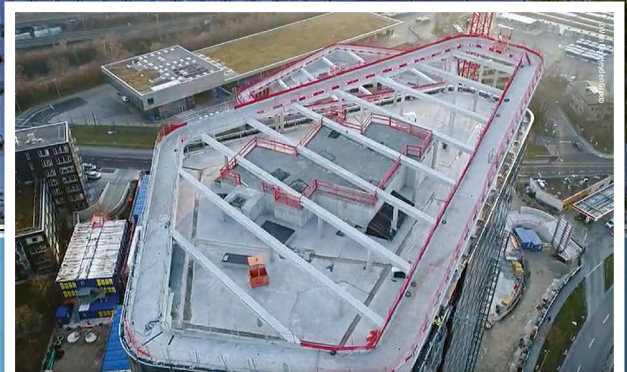
Steel beams were connected to the concrete trusses
