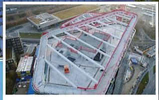
Steel beams were connected to the concrete trusses
