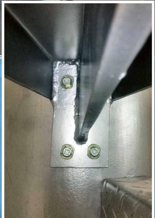
Hollo-Bolts were inserted into pre-drilled holes
