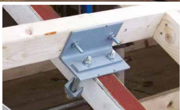
Purlin support cleat secured to existing RSA
