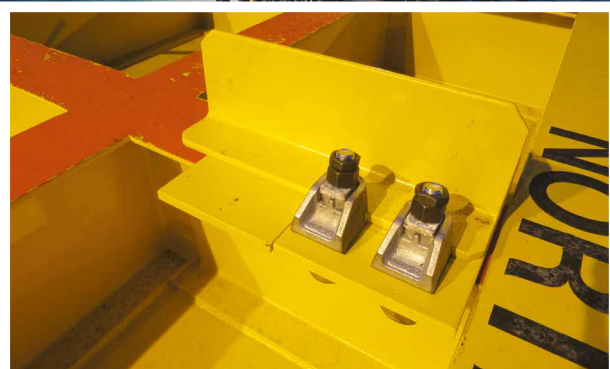
Type AF girder clamps securing the framework
