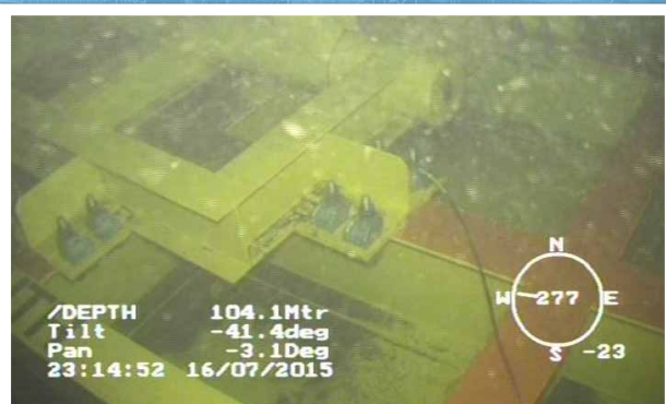
Base support frame in position on the seabed
